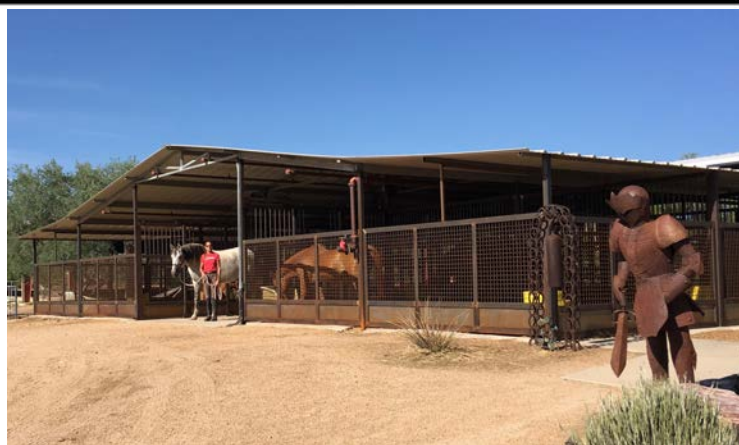
Front view of the newly renovated eight stall Camelot barn.
